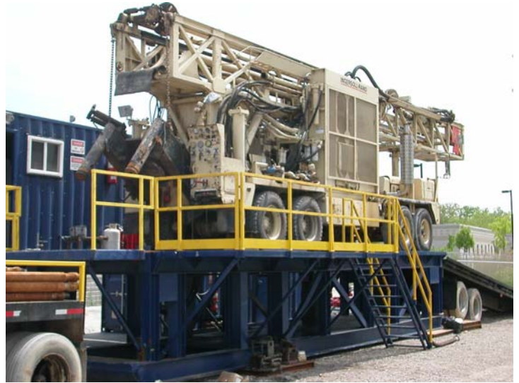
Rotary Drill Rig Setting Up on City of Windsor Property, May 2007.
