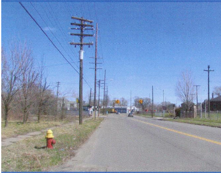
Existing Conditions - Looking North along Jefferson Avenue
