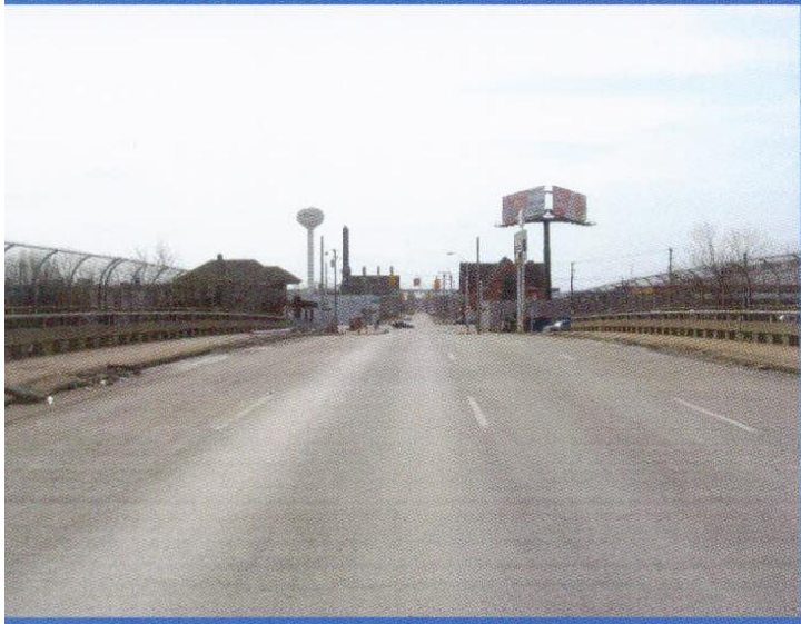
Existing Conditions - Looking East along Dragoon Street
