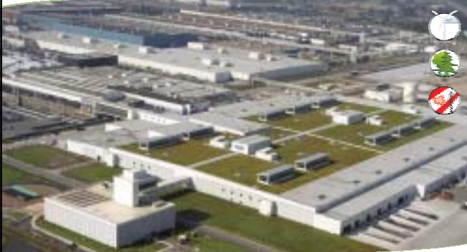
Example of Extensive Green Roofs
