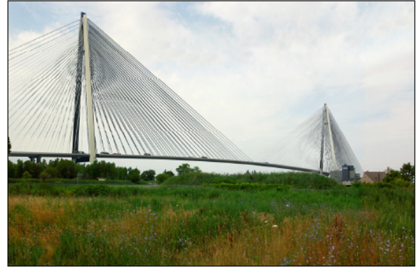
Cable-stayed bridge (illustration only)
