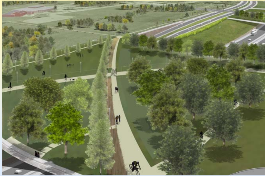
Aerial view of Oakwood short tunnel deck looking east
