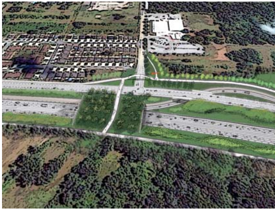
Aerial view of Pulford Street short tunnel looking northeast
