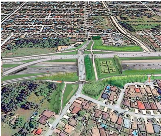
Aerial view of Grand Marais short tunnel looking northeast
