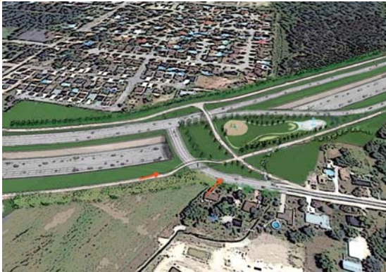
Aerial view of Huron Church Line short tunnel looking east
