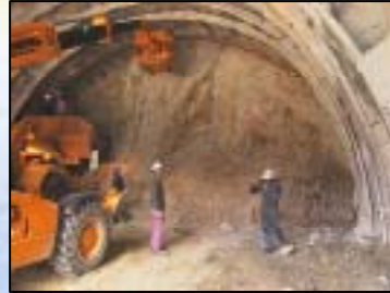
Soft Ground Tunneling
