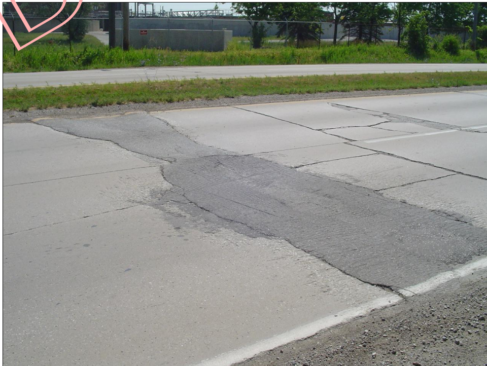
Photo 38 – Ojibway Parkway - north of E.C. Row Expressway
