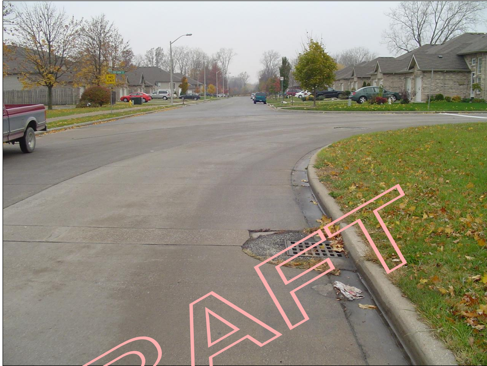
Photo 23 – Spring Garden Road - looking west
