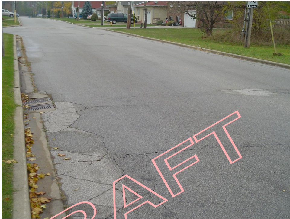
Photo 21 – Lambton Street - looking west
