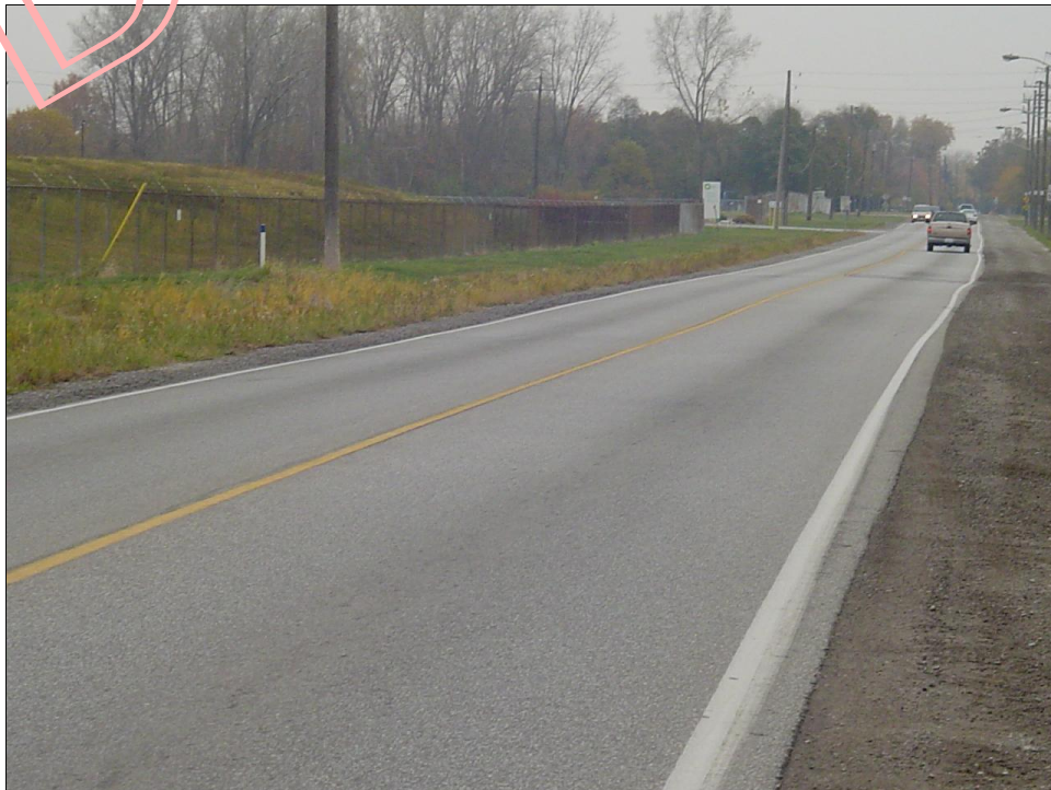
Photo 32 – Matchette Road – north of E.C. Row Expressway – looking north
