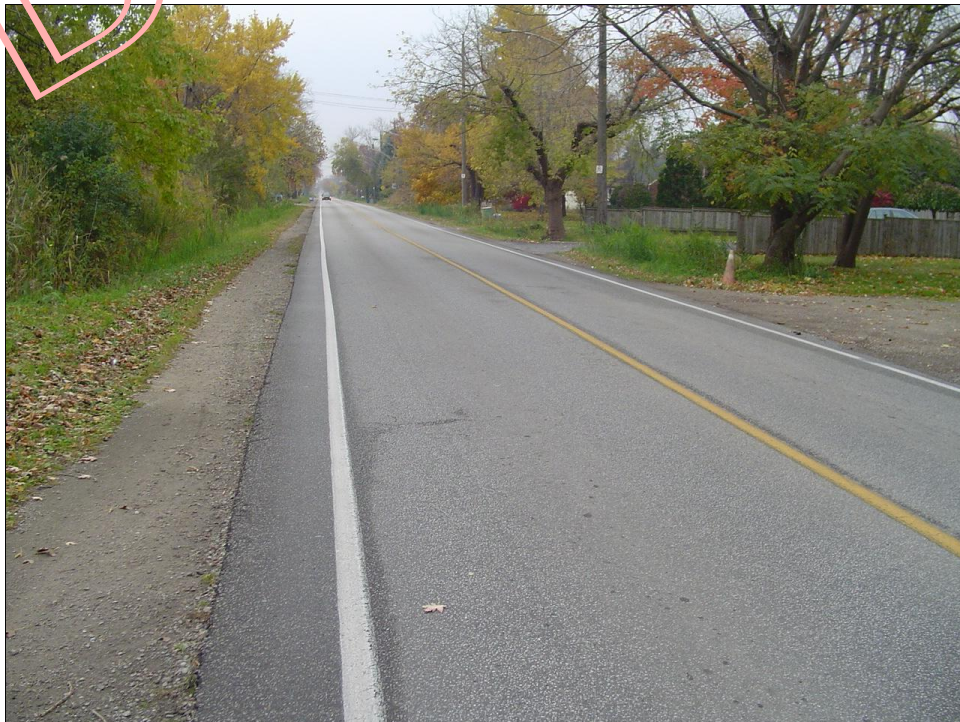
Photo 26 – Malden Road - south of E.C. Row Expressway - looking south
