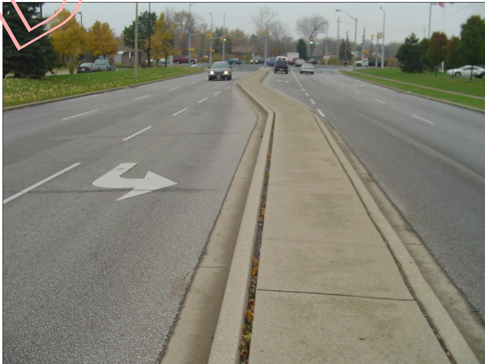
Photo 8 – Sandwich Parkway - looking north.
