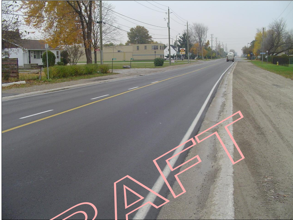
Photo 3 – Howard Avenue - south of Talbot Line - looking south.
