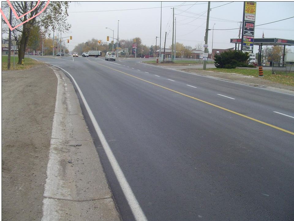
Photo 4 – Howard Avenue - south of Talbot Line - looking north.
