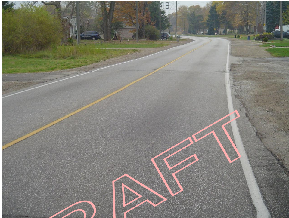
Photo 35 – Matchette Road – south of E.C. Row Expressway – looking south
