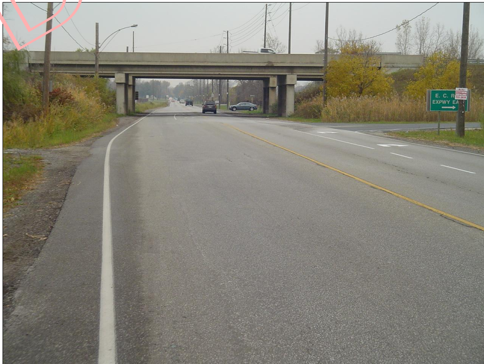
Photo 34 – Matchette Road – south of E.C. Row Expressway – looking north
