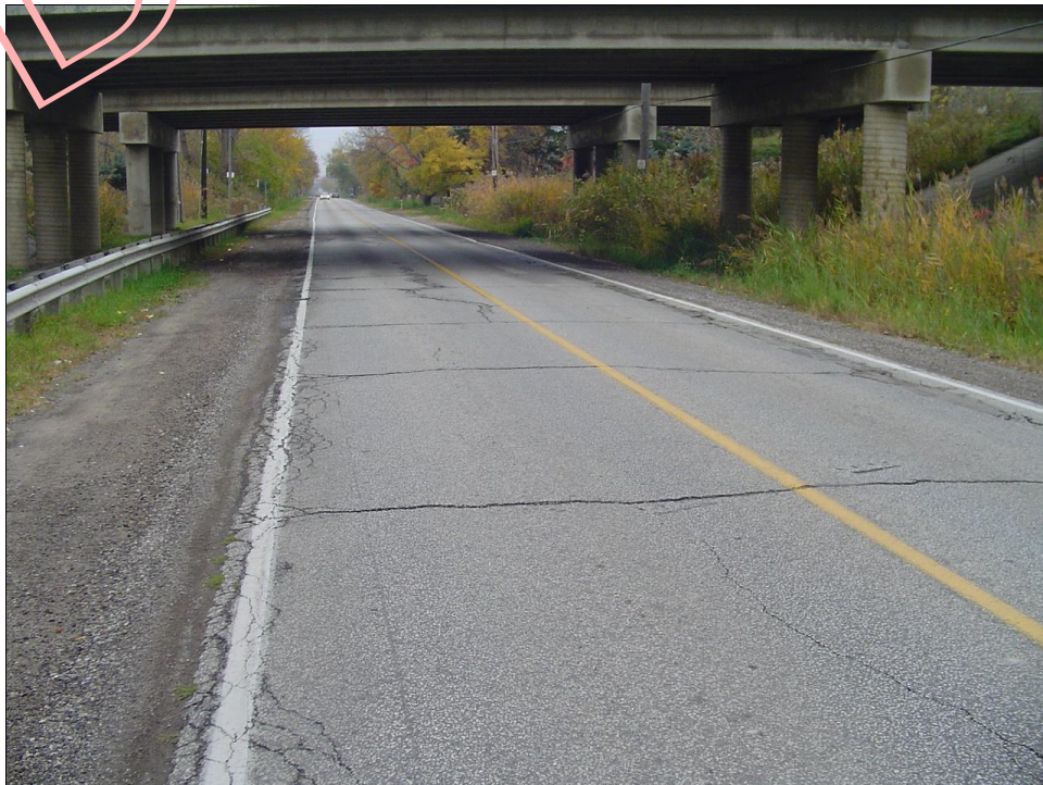
Photo 28– Malden Road - north of E.C. Row Expressway - looking south
