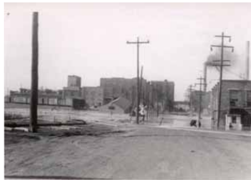
Photo 4. Looking west from near wells #20 and #4, south of liquid chlorine building, showing loss of high compressor building (middle ground) and shed 102b (background).
