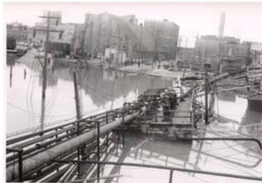
Photo 3. Looking west from between wells #20 and #14 on liquid chlorine building showing loss of chlorine pump building.
