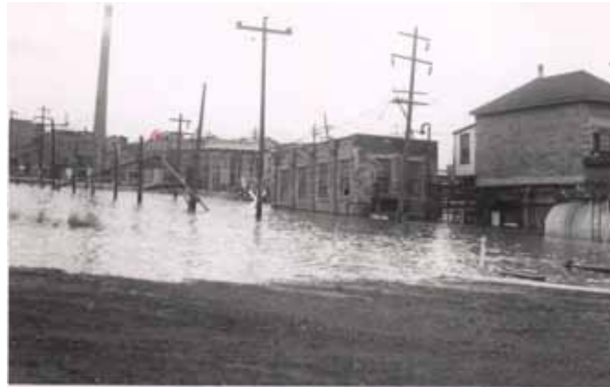
Photo 2. Looking west-northwest from between wells #10 and #20, in present open field showing loss of high compressor building (centre).
