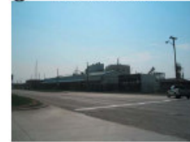
⑧ Detroit Water Treatment Plant
