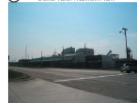
⑧ Detroit Water Treatment Plant
