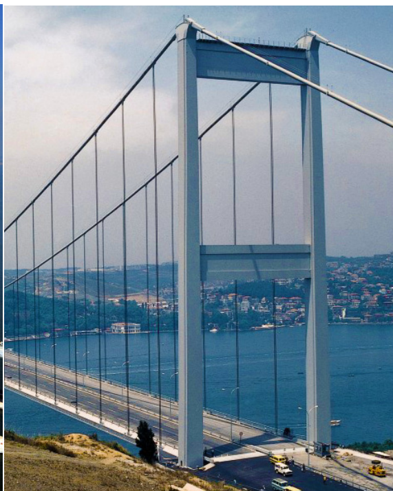
FATIH SULTAN MAHMET BRIDGE | IHI Inc.
