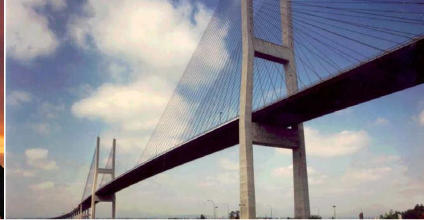
ANNACIS BRIDGE | PCL Civil Constructors, Inc.
