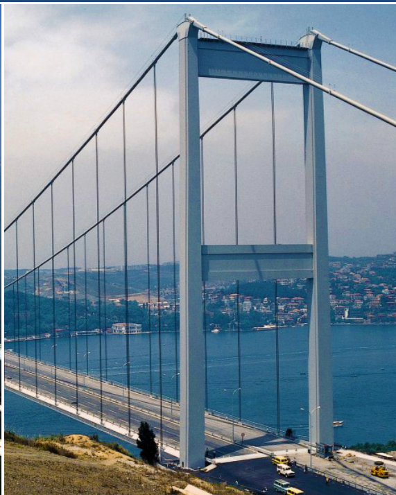
FATIH SULTAN MAHMET BRIDGE | IHI Inc.
