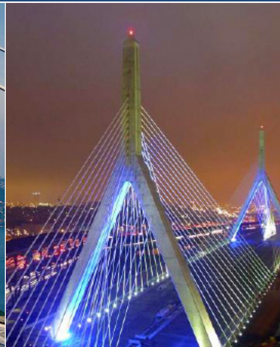
LEONARD P. ZAKIM BRIDGE | Parsons Brinckerhoff
