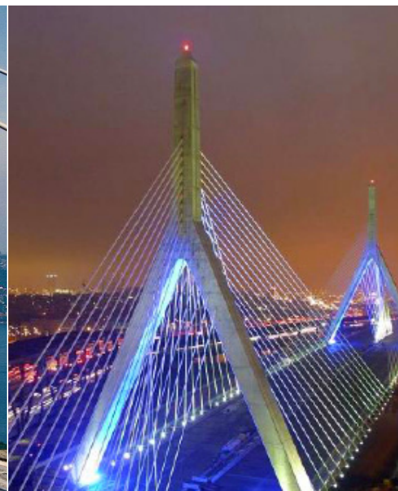
LEONARD P. ZAKIM BRIDGE | Parsons Brinckerhoff
