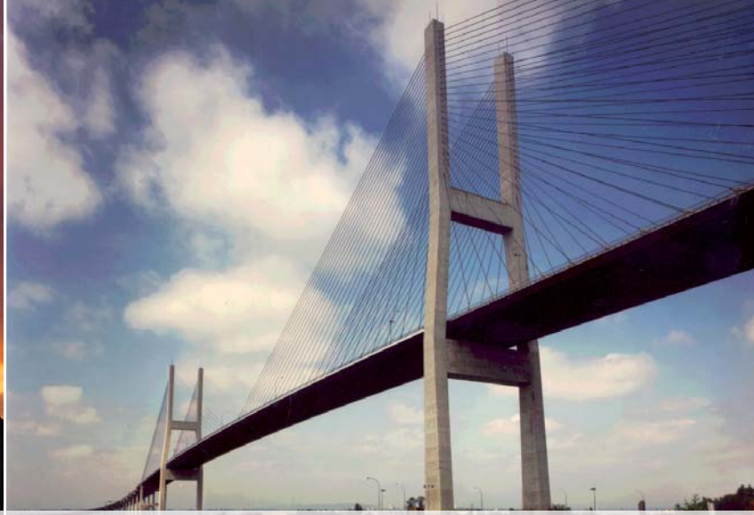
ANNACIS BRIDGE | PCL Civil Constructors, Inc.
