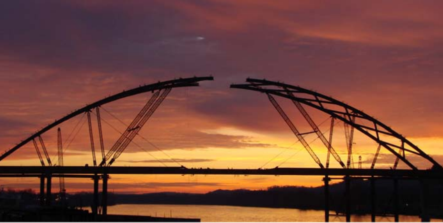
BLANNERHASSETT BRIDGE | Walsh Construction Company
