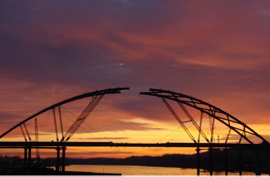
BLANNERHASSETT BRIDGE | Walsh Construction Company
