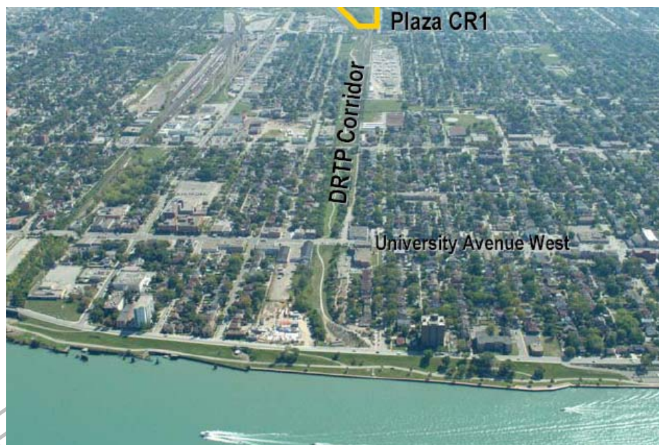
EXHIBIT 3.10: DRTP CORRIDOR – FROM DETROIT RIVER LOOKING SOUTH.
